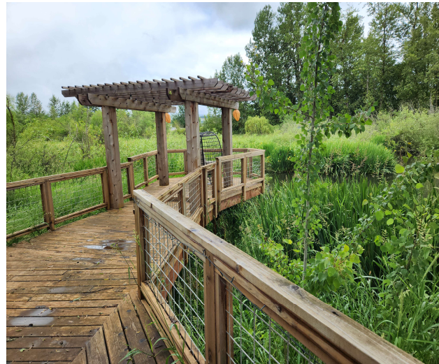
Encroachment into PEMC wetlands
